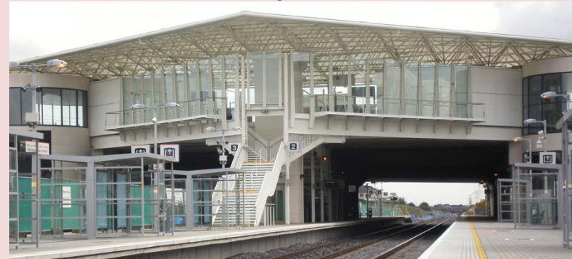
A space frame at Parkwest/Cherry Orchard Train Station
